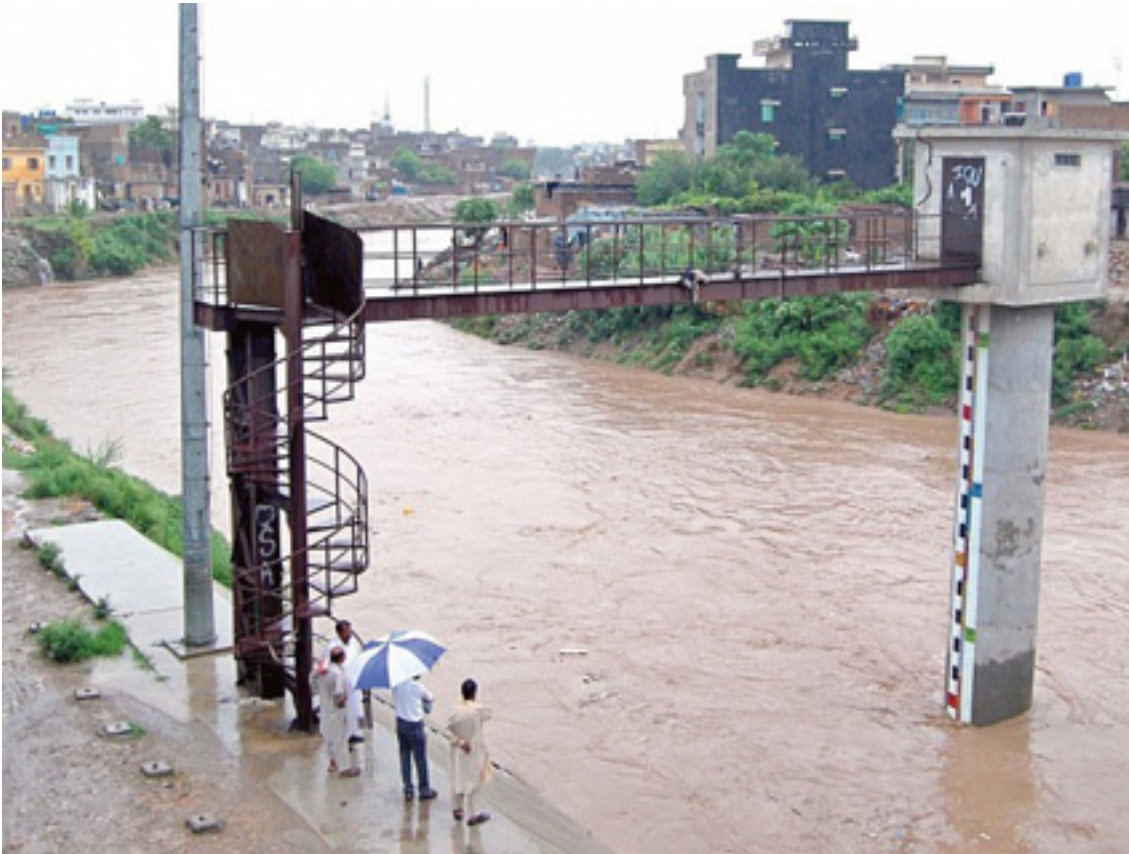
Flood warning station
