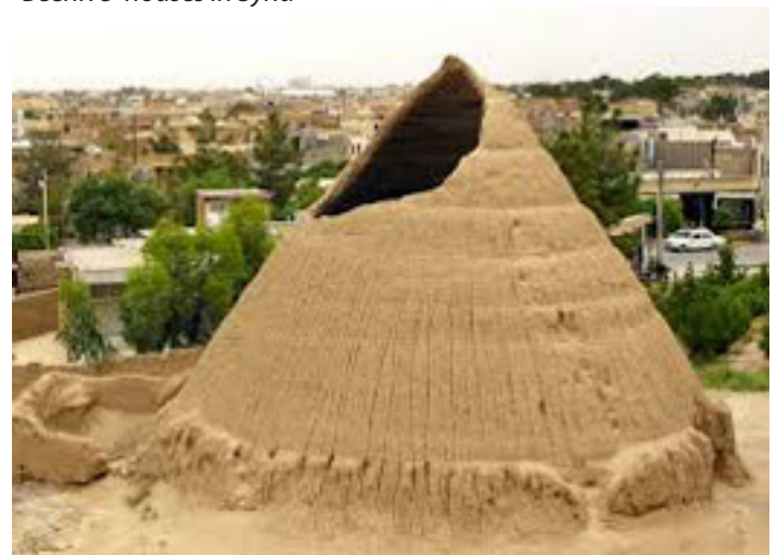
Iran's ancient ice houses which could keep ice frozen in deep cellars throughout the year
