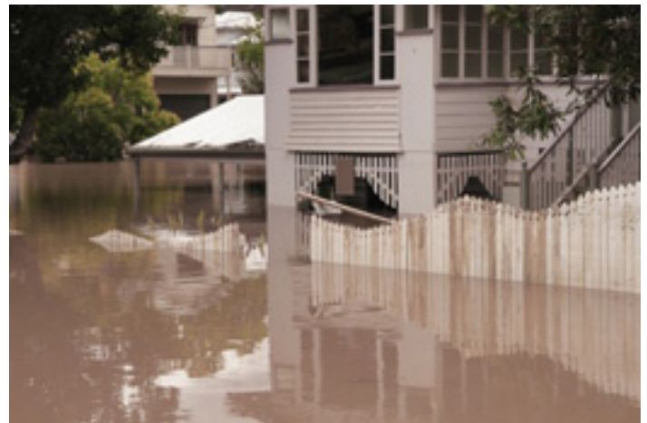
A "Queenslander" during flood season – the house itself sits high above the flood waters
